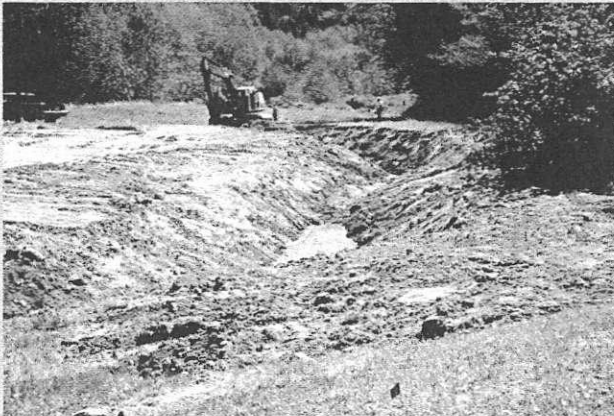
Construction phase of Prairie Creek Coho project
