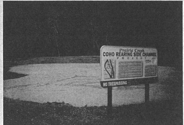
Completed Prairie Creek Coho project demonstrates what can be accomplished with determination and funding
