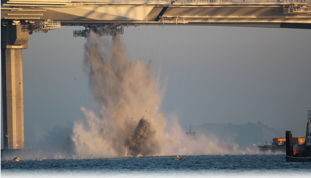
Staff wrote an incidental take permit amendment that would ensure the environmental effects from the implosion of pier E3 (San Francisco Bay Bridge) were monitored and that appropriate mitigation actions were identified.
