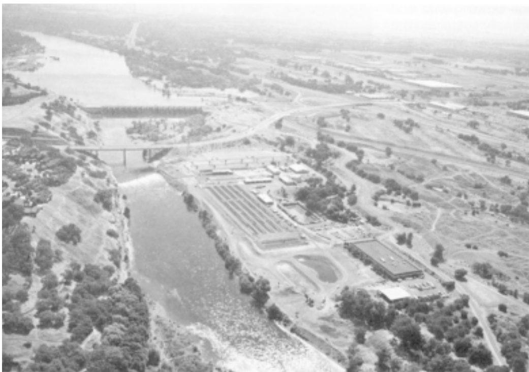
PHOTO: BUREAU OF RECLAMATION
