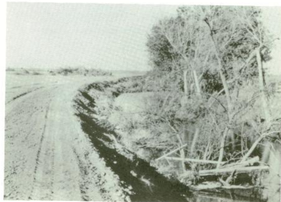
Note silt and debris in creek.
