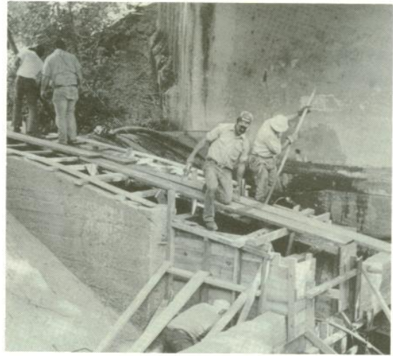
Members of the North Bay Chapter of Trout Unlimited pour concrete during the restoration of a deteriorated fish ladder on Corte Madera Creek, Marin County.
