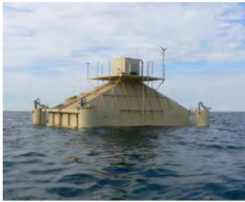
Oscillating water column device: Oceanlinx.
