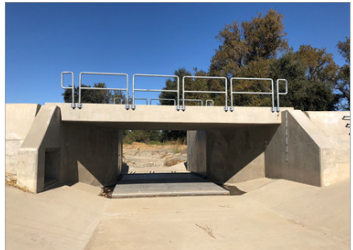
Fremont Weir fish ladder in 1965 (top) and 2018 (bottom). The new fish ladder provides much improved passage for adult winter-run Chinook salmon to return to the Sacramento River from the Yolo Bypass. Photos: U.S. Bureau of Reclamation.
